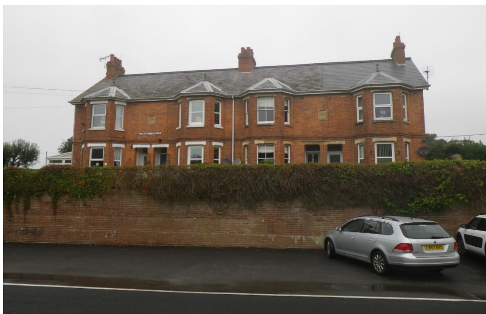
Standen Terrace No1 is on the left
